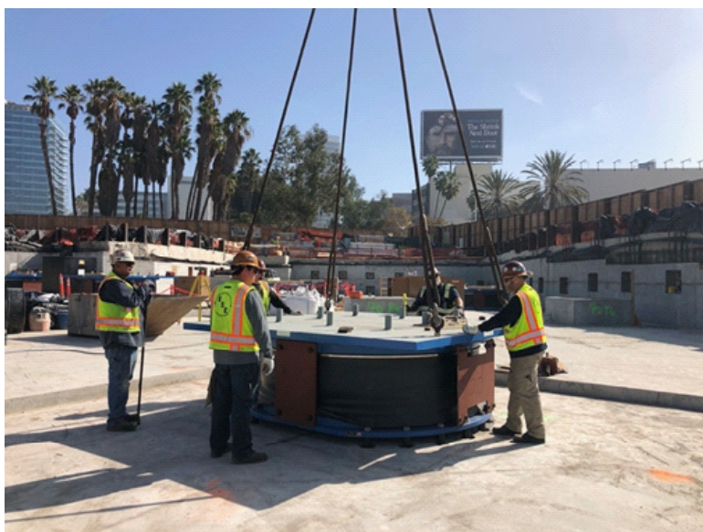
Figure 8: Isolation bearings at EPS' factory (left) and during installation on site (right).
